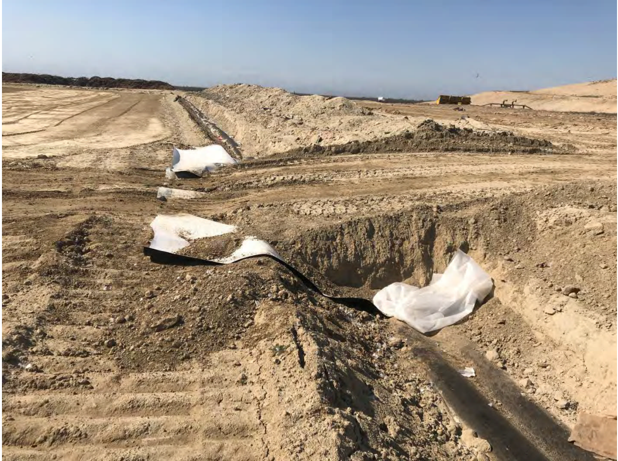
Figure 2. Method of Electrically Isolating Access Roads
