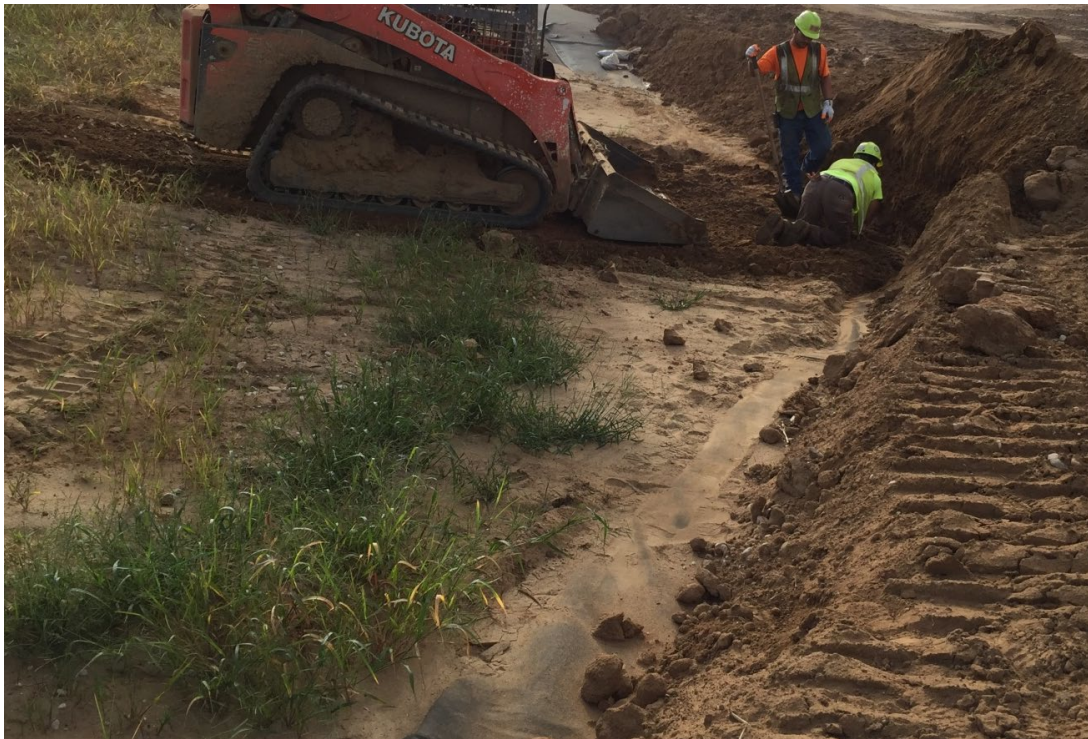
Figure 2. Excavation of Access Road to Survey Area.
